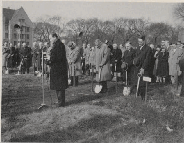
Delivered by Dean Walter Harrelson of the University of Chicago Divinity School at the groundbreaking for the new Law School Building.
